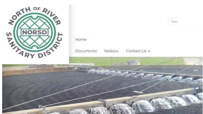
NORS D wastewater treatment plant Picture courtesy NORSD website
